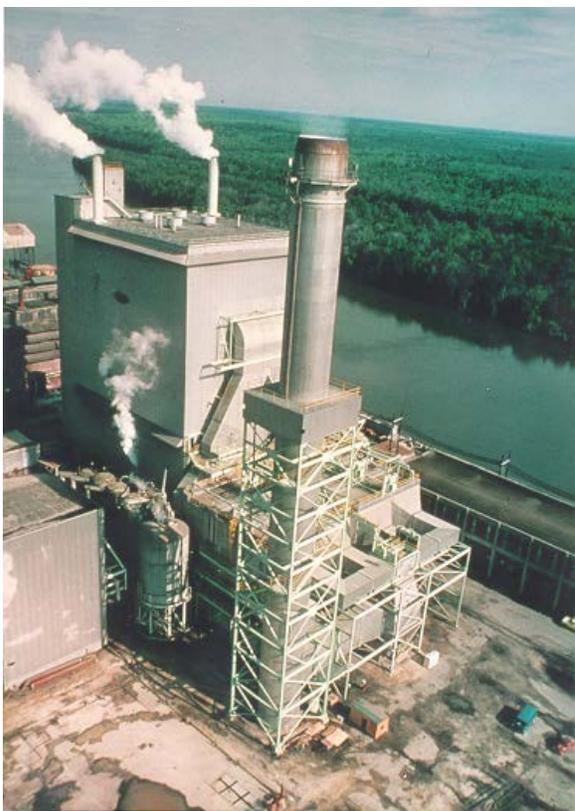
**Figure 10.** Black Liquor Recovery Boiler (BRLB)
