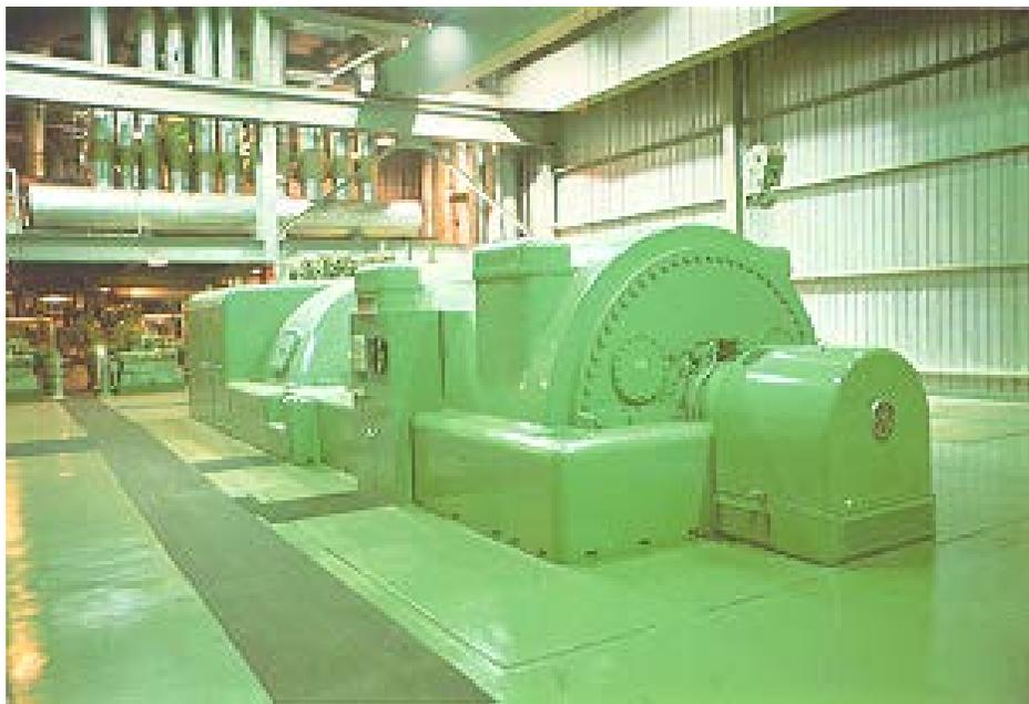
**Figure 15.** Steam Turbine-Generator
